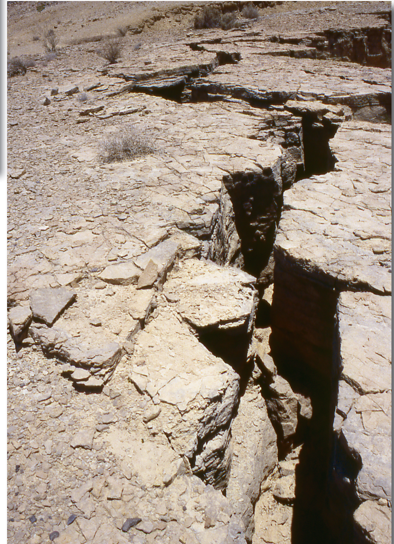
Fig. 57: Dramatic cracks at the limestone beds at the rim of Makhtesh Ramon, near the Visitors Center (Mazor)
